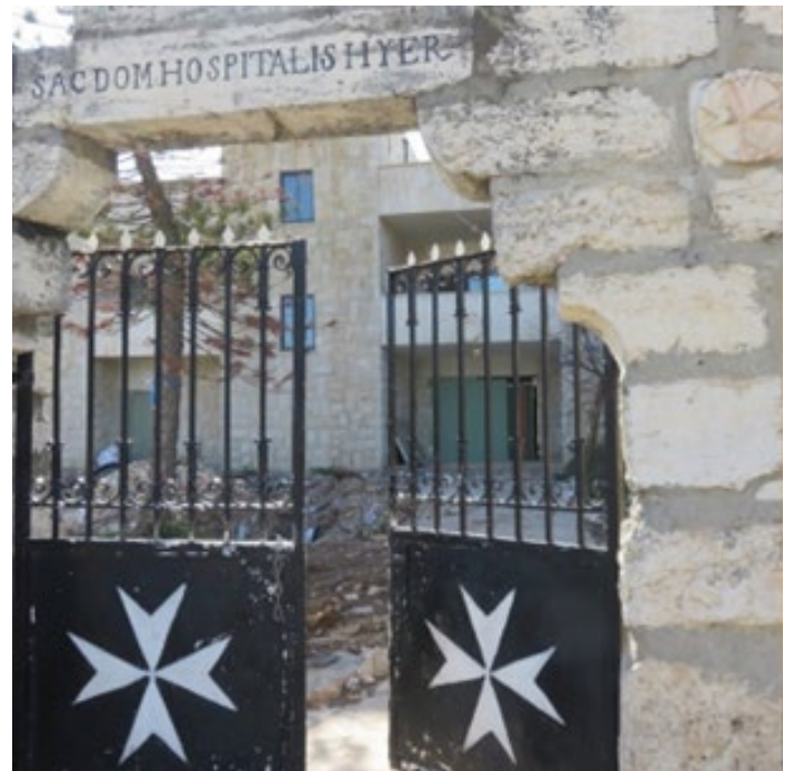
The original gates of the hospital remain, now leading to the modern buildings of the Foundation Pro Tantur within the University of Notre Dame. © photograph by the author.
