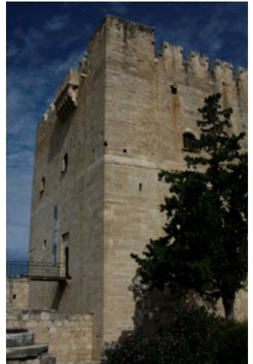
Kolossi Castle. This fortress was originally constructed by the Knights of St John in 1210. © photograph by B. Caslake.
